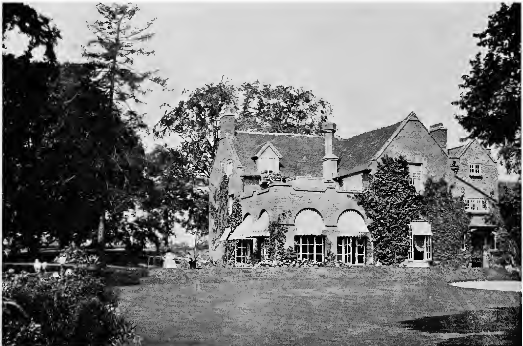
THE LOWE, WELLESBOURNE, WARWICK. ALTERED AND ADDED TO FOR MRS. NICOL. THE MATERIALS ARE RED BRICK AND RED TILES CHOSEN TO MATCH THE OLD PARTS OF THE BUILDING
