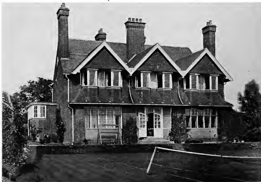
HOUSE AT STANMORE IN RED BRICKS, WITH A ROOFING OF SAND-FACED TILES. VIEW FROM THE GARDEN
