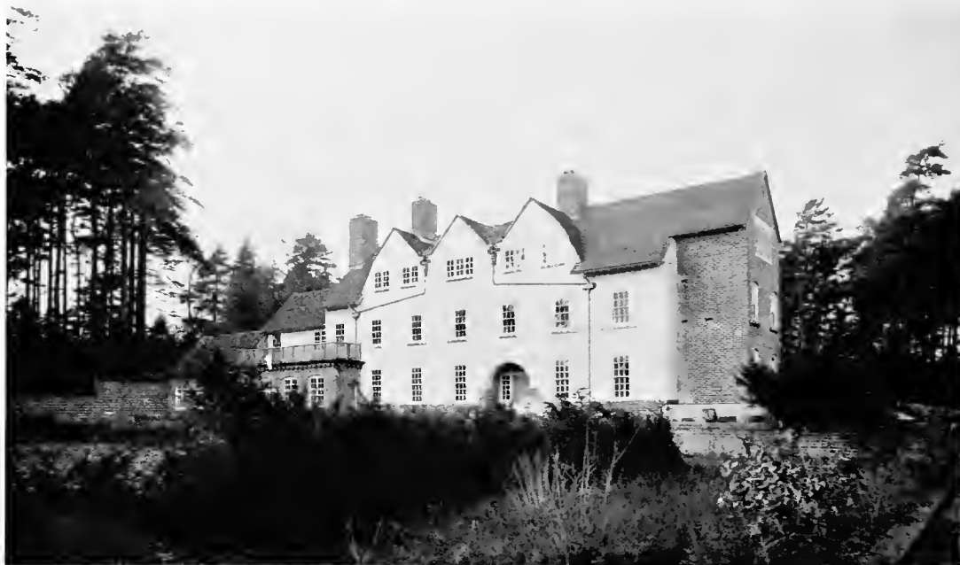
HOUSE (IN COURSE OF CONSTRUCTION) AT GRAFFHAM, NEAR PETWORTH, SUSSEX. BUILT OF BROWN LOCAL STOCKS IN PART ROUGHCASTED, AND ROOFED WITH PLAIN RED TILES
