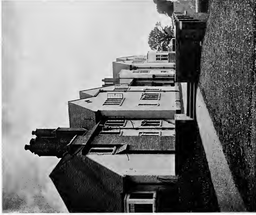
GREYSTOKE, NEAR WARWICK, BUILT OF BRICK AND ROUGHCAST, WITH SMALL RED BRICK FACINGS TO THE CHIMNEYS AND PLINTH, THE ROOFING OF HAND-MADE RED TILES
