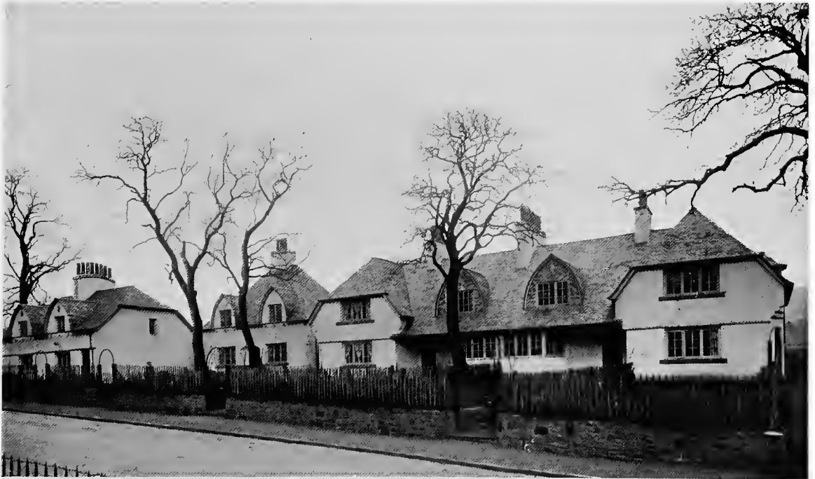
GROUP OF COTTAGES AT COLINTON, MIDLOTHIAN. BUILT OF STONE HARLED AND WHITEWASHED, AND ROOFED WITH SCOTCH SLATES
