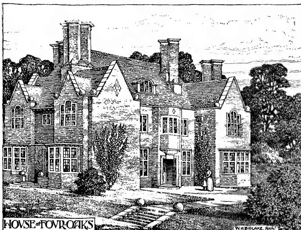
HOUSE AT FOUR OAKS, NEAR BIRMINGHAM. BUILT OF RED SANDSTOCK BRICKS, THE ROOFING OF RED TILES
