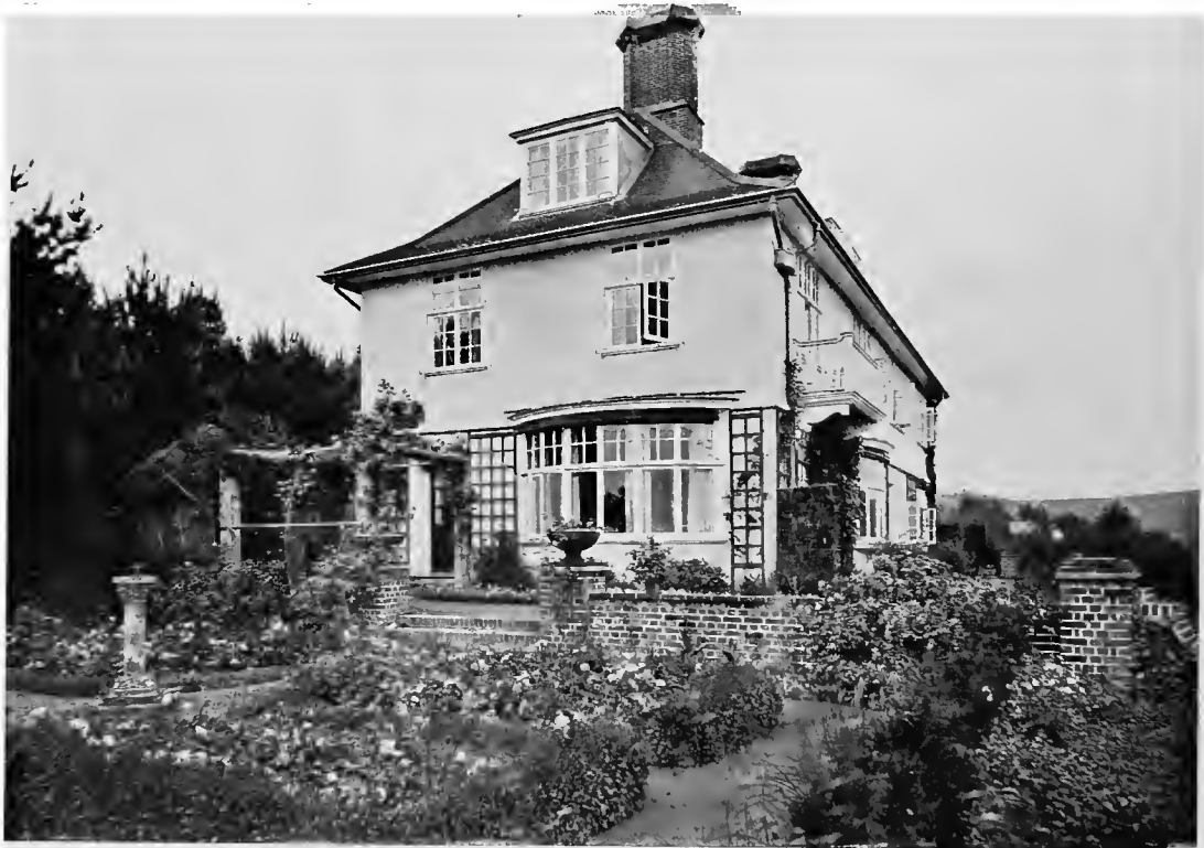
HOUSE ON THE HINDHEAD, BUILT OF BRICK AND ROUGHCAST, WITH RED BRICK CHIMNEYS AND A ROOFING OF BROWN TILES; THE WOODWORK IS PAINTED WHITE THE DOORS AND THE TRELLIS ARE GREEN
