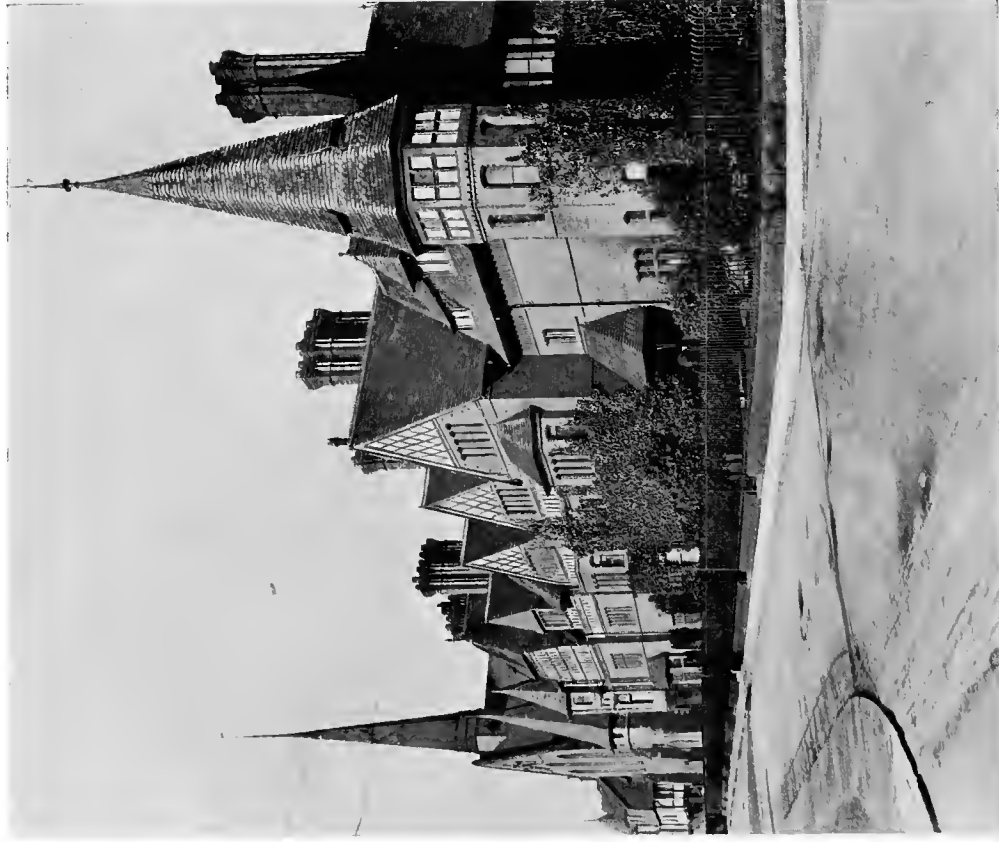
HOUSES AND A CHAPEL IN GROSVENOR ROAD, CHESTER, BUILT OF RUABON BRICK, WITH MOULDED BRICK WINDOWS, ETC., AND THE ROOFING OF BROWN TILES
