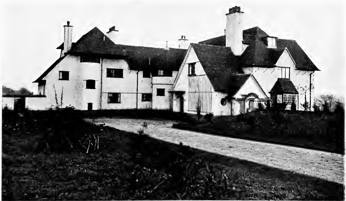
WALWOOD, SURREY, THE FORECOURT ENTRANCE. THE HOUSE IS OF BRICK AND ROUGHCAST WITH A BASE OF RED BRICK AND A ROOFING OF RED TILES. THE WINDOWS ARE LEADED CASEMENTS
