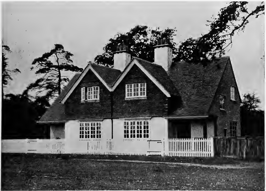
TWO COTTAGES AT RIPLEY, IN SURREY, COSTING £585 THE PAIR. MATERIALS: ROUGHCAST AND LOCAL TILES
