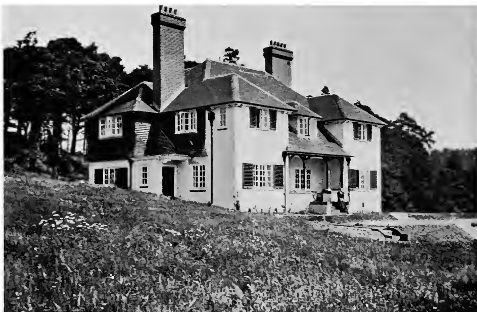
HOUSE AT HEYSHOTT, NEAR MIDHURST, COMPLETE COST £1337, INCLUDING WOOD AND COAL SHED, GARDEN TOOL HOUSE, ETC. MATERIALS: ROUGHCAST. RED BRICKS, TILE HANGING, TILE ROOF
