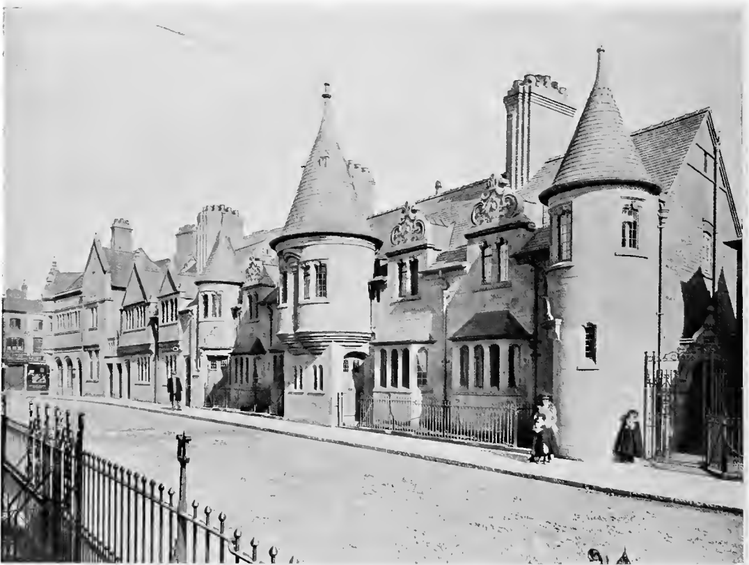
COTTAGES, BATH STREET, CHESTER. BUILT OF LOCAL RED SANDSTONE, WITH RUABON BRICK CHIMNEYS AND GREY-SLATED ROOFS
