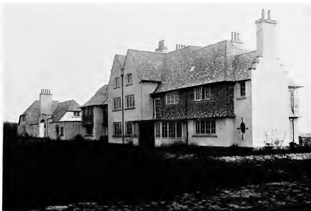
HOUSE AT NORTH BERWICK, VIEW FROM THE S.W. BUILT OF LOCAL WHINSTONE HARLED AND WHITEWASHED, WITH SLATE-HANGING AND ROOFS OF SCOTCH SLATES
