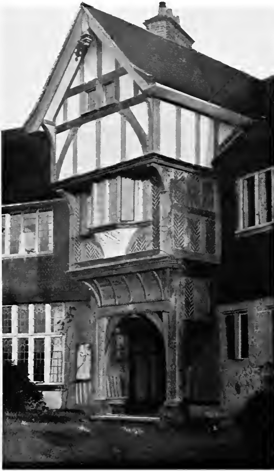
HOUSE ON THE HINDHEAD, SURREY, VIEW OF THE PORCH, A PIECE OF TIMBER CONSTRUCTION ALL IN OAK, FILLED IN WITH BRICKWORK AND PLASTER WHITEWASHED
