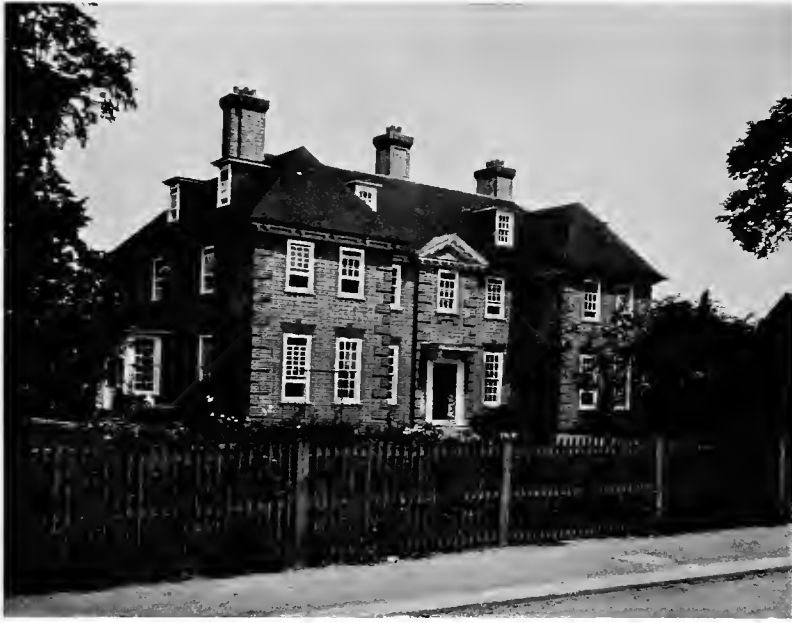
HOUSE AT REIGATE, SURREY. RED BRICK QUOINS, THE FILLING OF DARKER BRICKS FROM HOLDEN CRAWLEY, IN BERKSHIRE. THE CORNICE OF WOOD, THE ROOFS OF RED, SAND-FACED TILES
