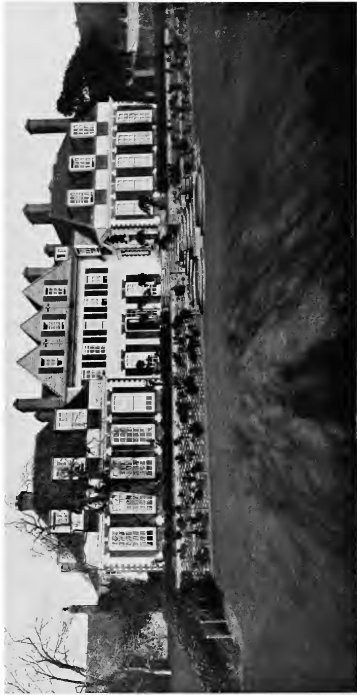
THE HOO, WILLINGDON, SUSSEX, BELONGING TO ALEXANDER WEDDERBURN, ESQ. VIEW OF THE SOUTH ELEVATION. THE HOUSE IS ROOFED WITH RED TILES, THE WALLS ARE DINGED WITH LIME, THIN RED BRICKS ARE USED FOR THE CHIMNEYS AND THE DRESSINGS; THE BOARDING IN THE GABLES IS OF ELM
