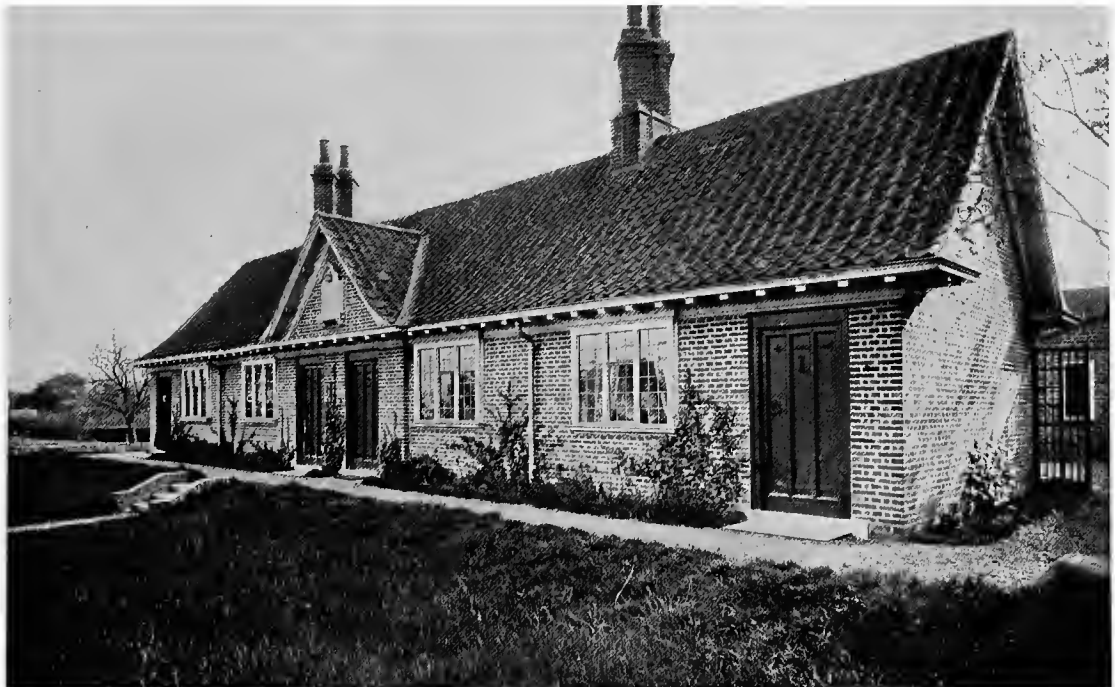
FOUR ALMSHOUSES AT WESLINGTON, YORKSHIRE, BUILT FOR LORD DERAMORE. MATERIALS: WALLS OF LOCAL BRICKS 2" THICK, THE ROOFING OF HAND-MADE PANTILES
