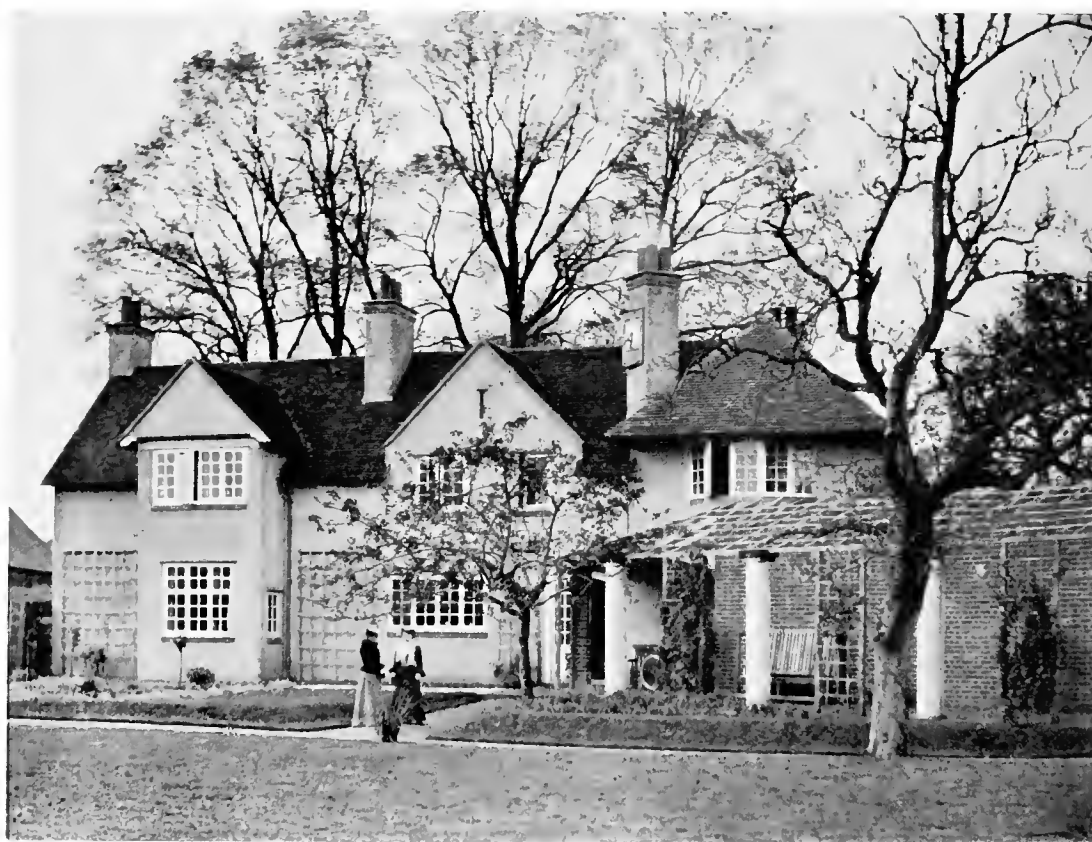
THE EYOT HOUSE, SONNING-ON-THAMES. BUILT OF LOCAL STOCKS ROUGHCASTED, AND ROOFED WITH PLAIN RED TILES
