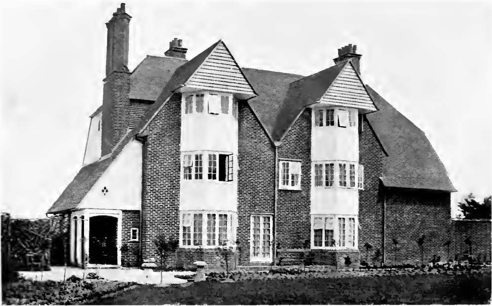
THE CROFT, WINCHFIELD. HANTS. VIEW TOWARDS THE LAWN, FACING S.W. MATERIALS: RED HAND-MADE BRICKS AND ROOFING TILES, ELM BOARDING TO GABLES, ROUGH WHITE PLASTER FOR THE BAYS, ETC.
