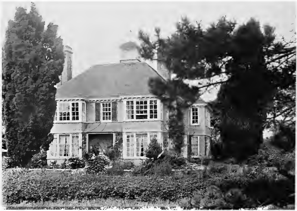
HOUSE AT RUSHMEN, NEAR IPSWICH. BUILT OF ROUGH BRICK AND OF ROUGHCAST COLOURED A RICH BUFF; THE ROOFING OF BROWN TILES, WHITE WOODWORK, GREEN SUN-SHUTTERS AND VERANDAH
