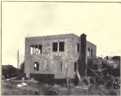
TILE HOUSE IN PROCESS OF CONSTRUCTION.
