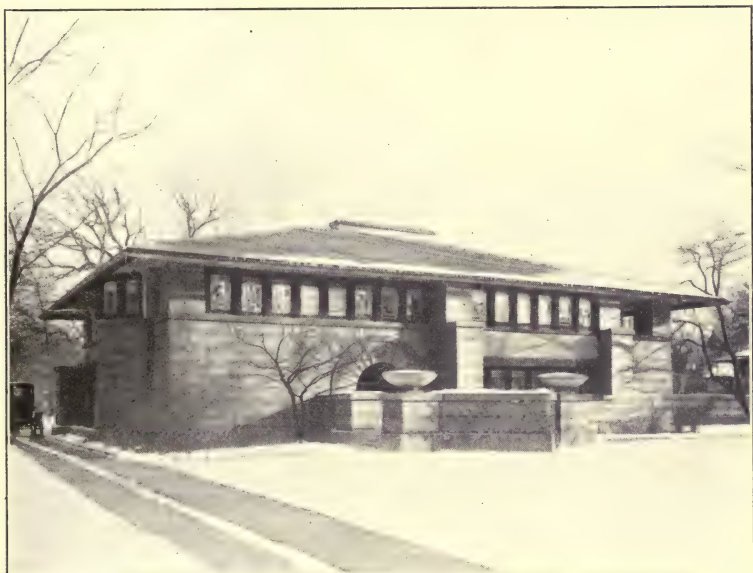
HOUSE FACED WITH PAVING BRICK.
