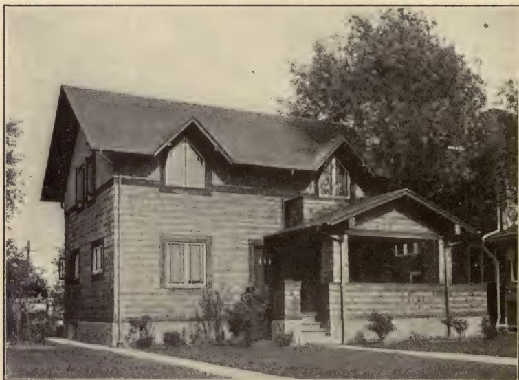
SHINGLES APPLIED WITH ALTERNATE WIDE AND NARROW COURSES.
