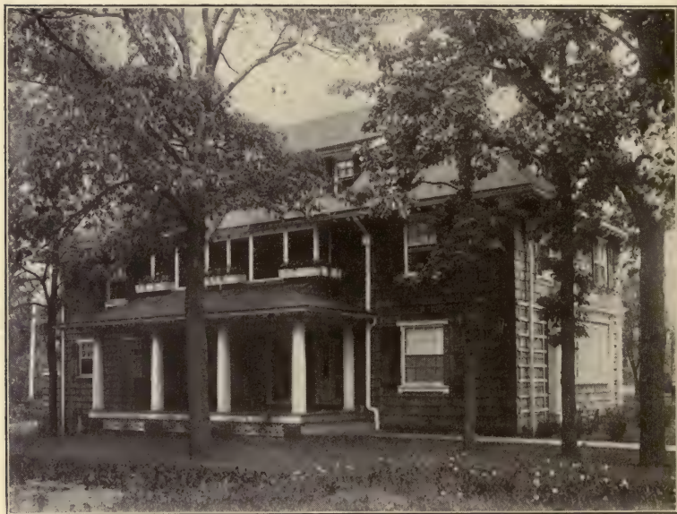
GALVANIZED IRON GUTTER AND CORNICE.
