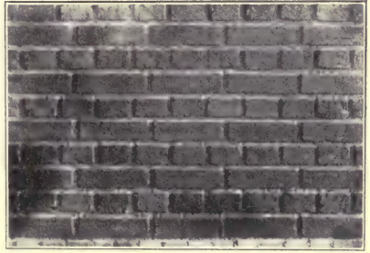
BRICKWORK LAID IN ENGLISH BOND.
