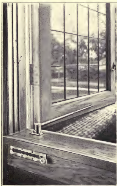
IMPROVED CASEMENT WINDOW ADJUSTER (OBVIATES OPENING SCREEN TO OPEN WINDOWS).
